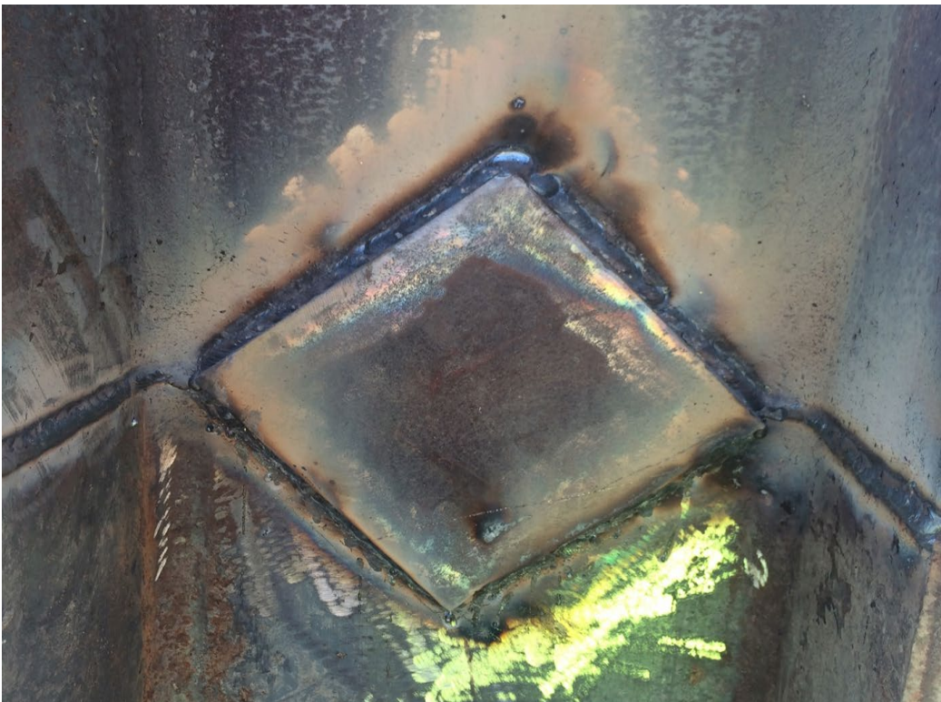
Completed backgouge and subsequent back side weld, as well as splice plate weld
