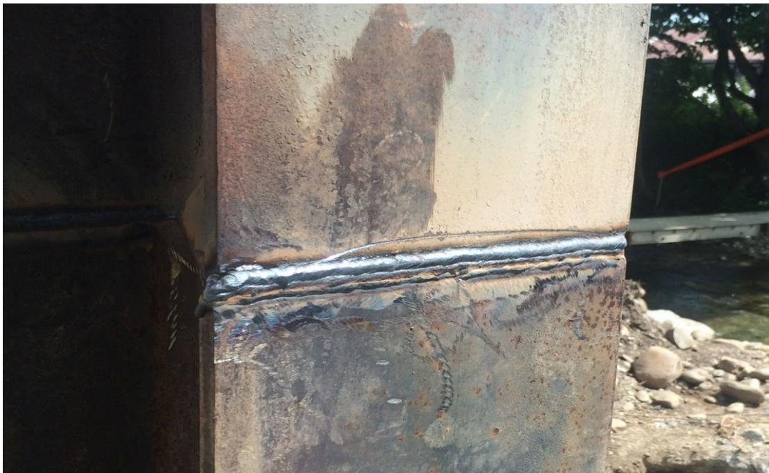
Completed outside of flange weld
