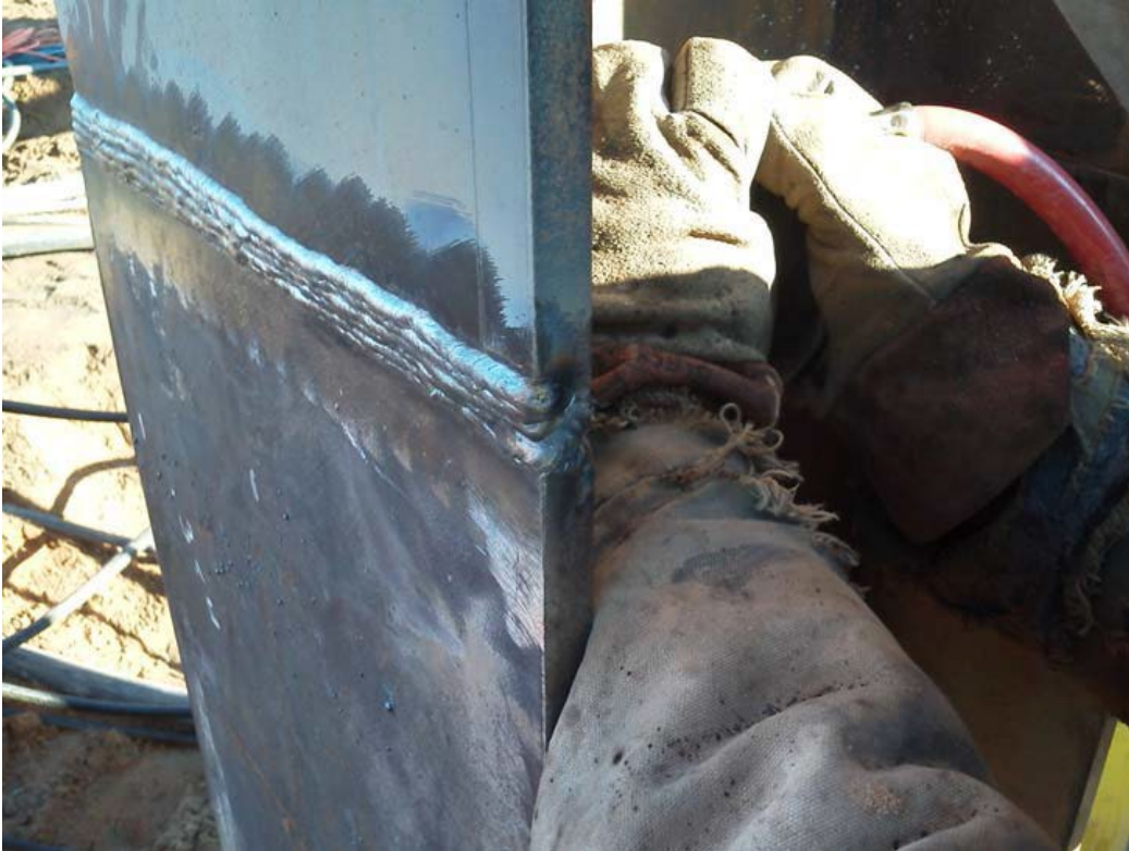
Back gouging to sound metal before welding the back side
